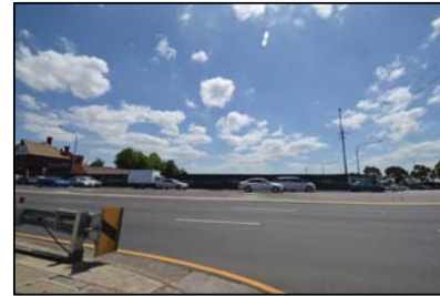
Figure 17: Partial view from the south-east corner of Hume Highway and Hoxton Park Road onto subject site (right) and part of the heritage item (left).
