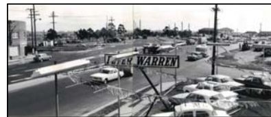
Figure 12: Corner of Hoxton Park Road and the Hume Highway at Liverpool in 1968 (Source: National Library of Australia: available at: http://trove.nla.gov.au/ , accessed 09.01.15)
