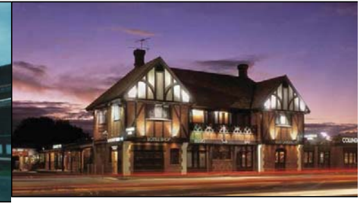
Figure 14: Primary façade of the Collingwood Hotel as it is today (Source: Google Maps and Photos, available at: https://www.google.com.au/maps/ , accessed 09.01.15)
