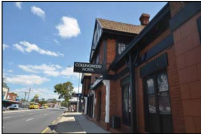
Figure 19: Close-up view onto façade of the heritage item Collingwood Inn Hotel at 321 Hume Highway, Liverpool, looking south, with recent single-storey extension in the forefront.
