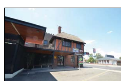
Figure 29: View onto the east corner of the south façade of the heritage-item, part of its primary significance, seen from the car park and northward bound traffic.
