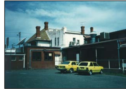
Figure 13: Colour photograph of the rear of Collingwood Hotel (west façade) as it appeared in 1991 (Source: National Library of Australia: available at: http://trove.nla.gov.au/ , accessed 09.01.15)
