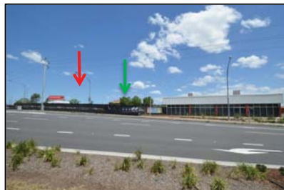
Figure 22: Location of subject site as seen from Hoxton Park Road, indicated by red arrow, and existing adjacent commercial building to the right. There are minimal views onto areas of less significance of the heritage item Collingwood Inn Hotel, indicated by the green arrow.
